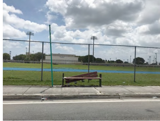
“Broken Bus Bench in the sun”
